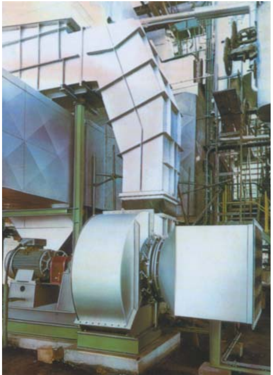
Centrifugal F. D. fan with inlet vane control I and inlet silencer. ▶
